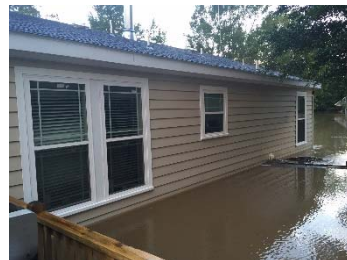
August 2016 – Louisiana Facility – 1000 Year Flood
