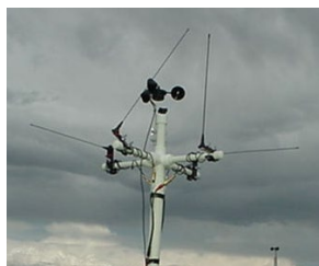
Ground Receiver and Antenna System
